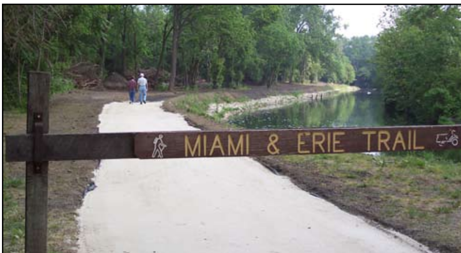
Section of the newly dedicated walkpath is still under construction.
