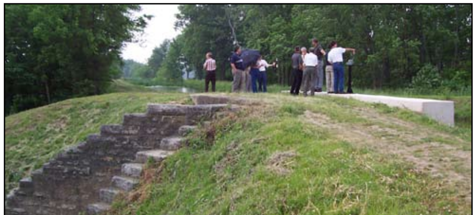
Ohio Water Advisory Council members at 6-Mile Creek Aqueduct.
