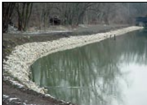
Stone walkway project near St. Marys.
