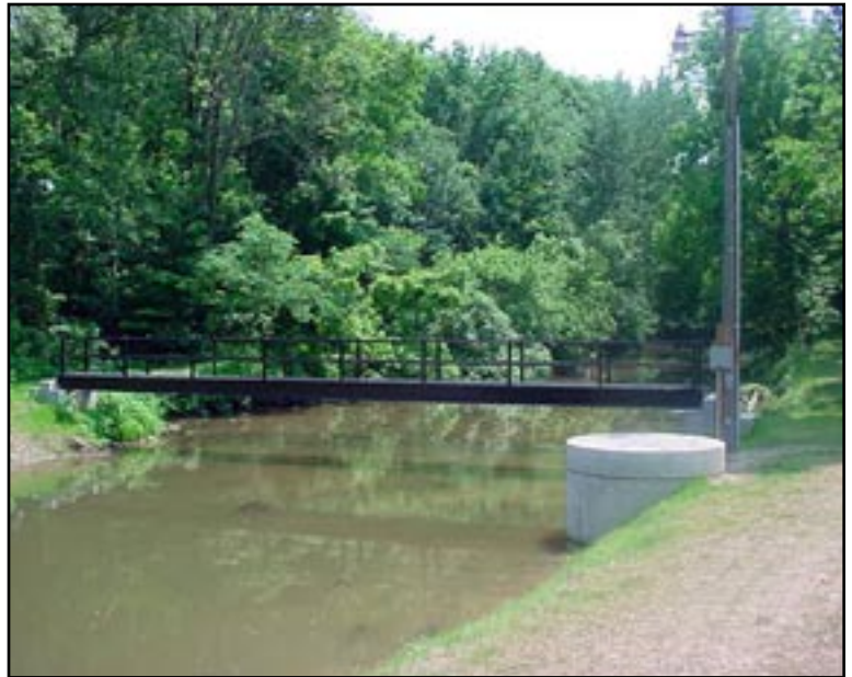
New foot bridge crossing the canal at 6-Mile Spillway.
