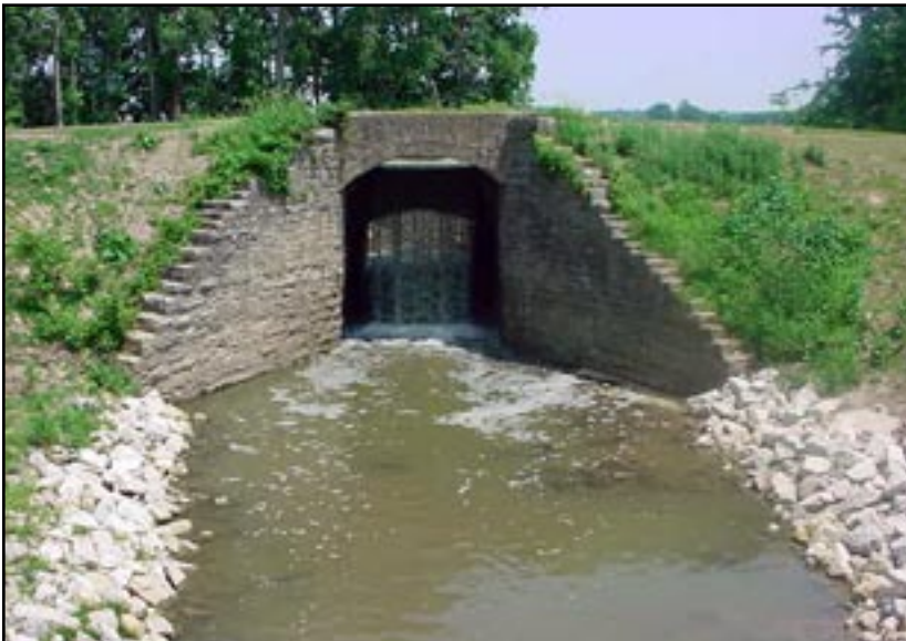
Renovations to the 6-Mile Spillway have been completed.
