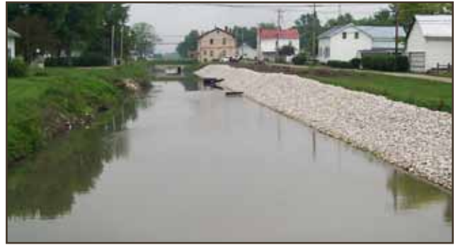
Work on the canal in the village of Minster.
