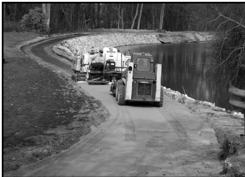
Lock 14 Towpath Trail under Construction Near Glynwood Road.
